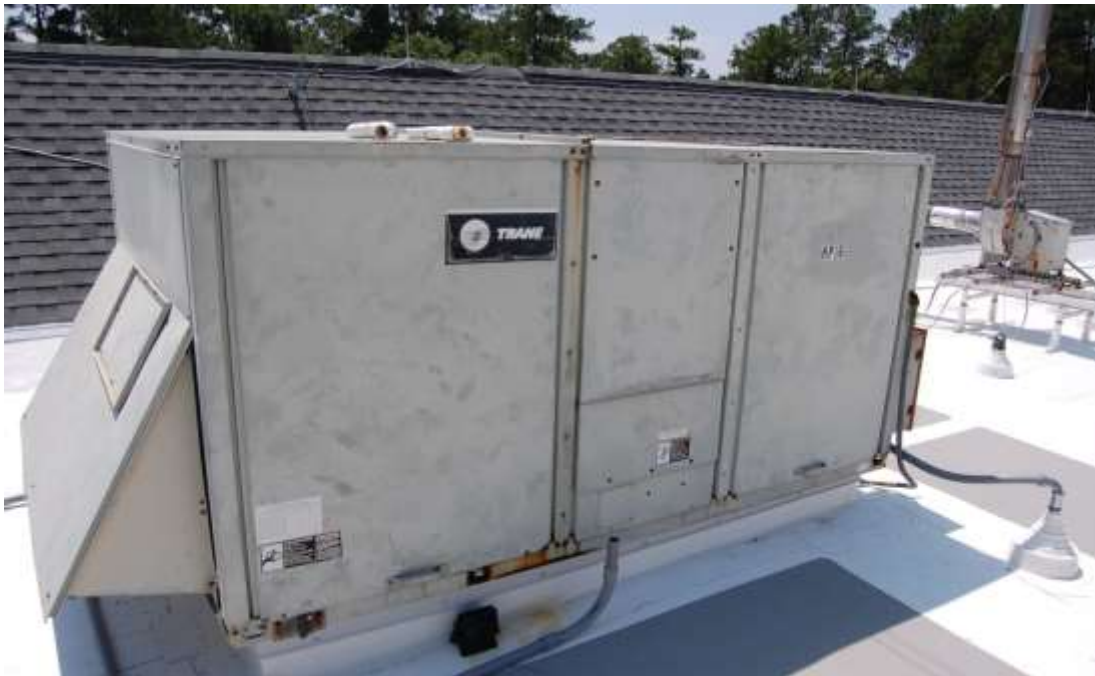
Existing 10 Ton HP #6 to be replaced
