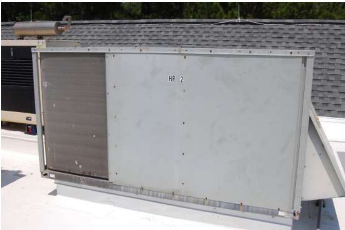
Existing 10 Ton HP #2 to be replaced
